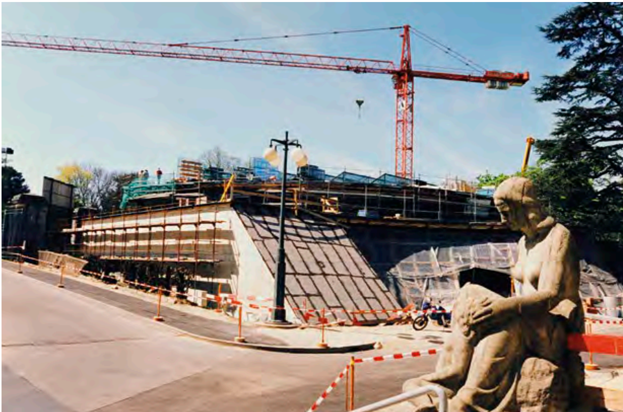
Construction of the Council Room to provide additional meeting space at the WTO's headquarters in Geneva.
