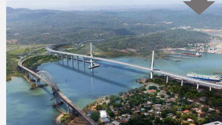
Panama Canal Fourth Bridge Project of CCCC
