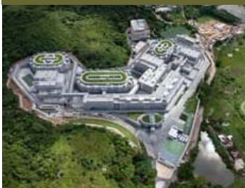
Yau Lee Curtain Wall and Steel Works
