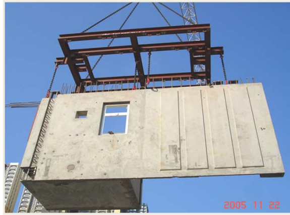
Precast Bathroom with noise barrier
